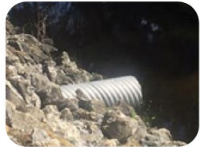
Outfall to River
