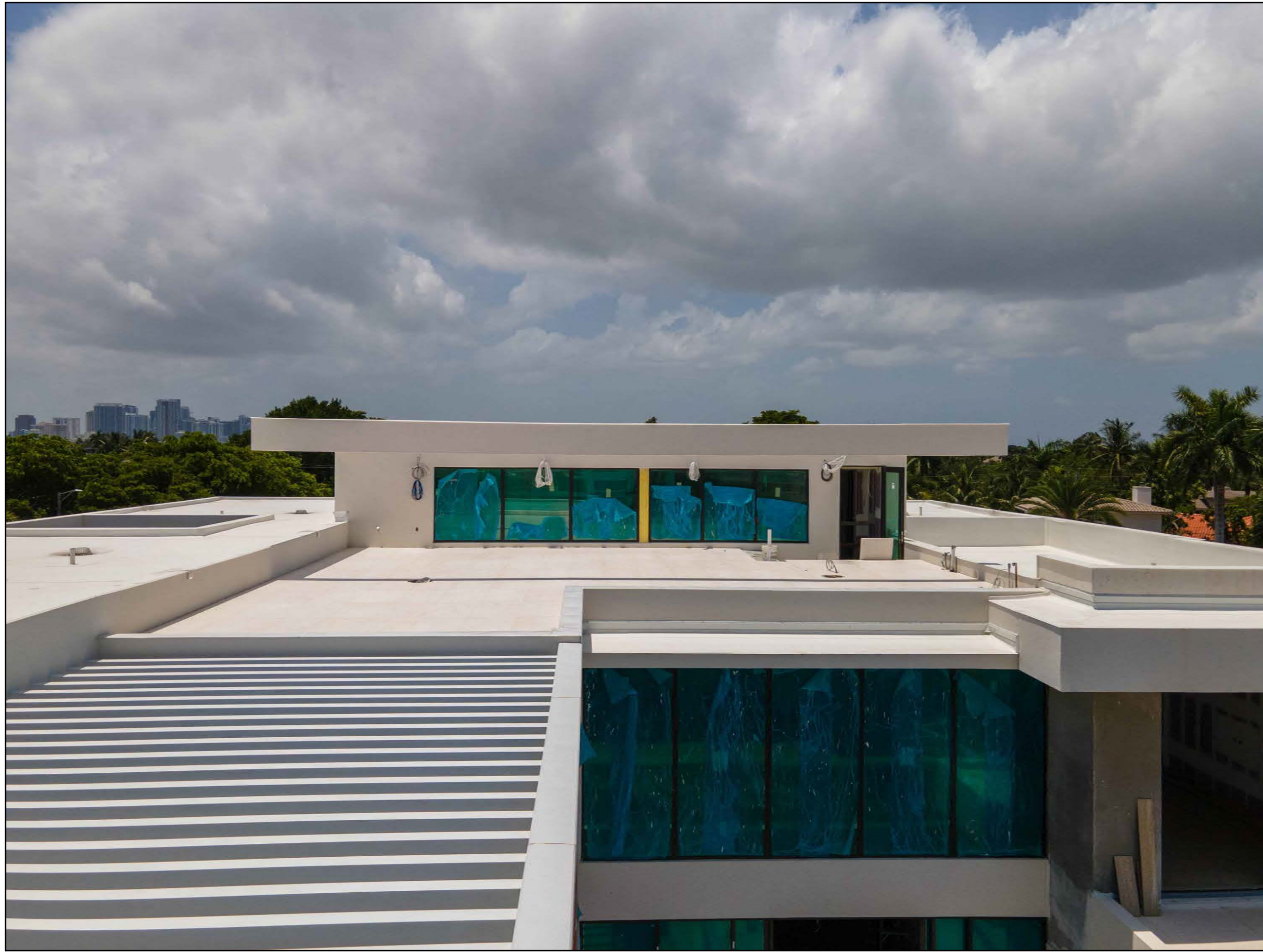
AERIAL VIEW #9: EAST SIDE, ROOFTOP REAR ELEVATION
