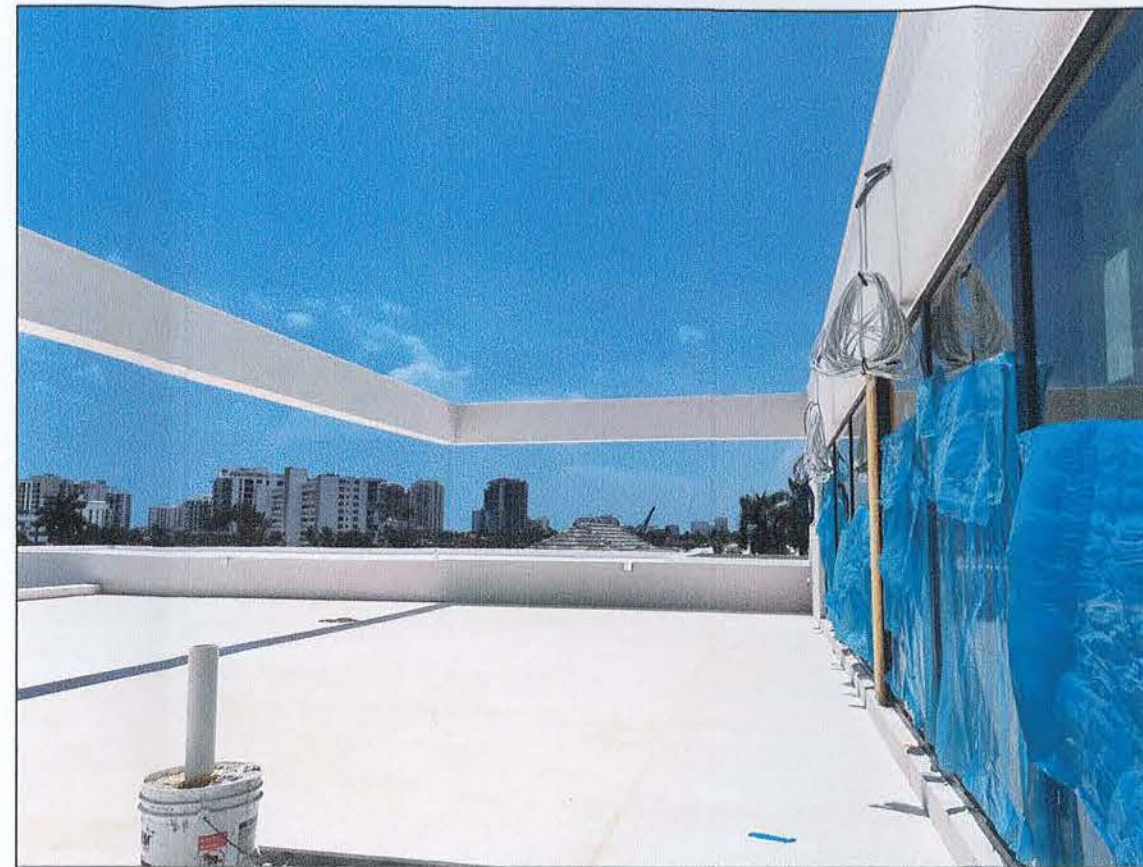
2 FIELD PHOTOS #2: ROOFTOP BEAMS FACING EAST
