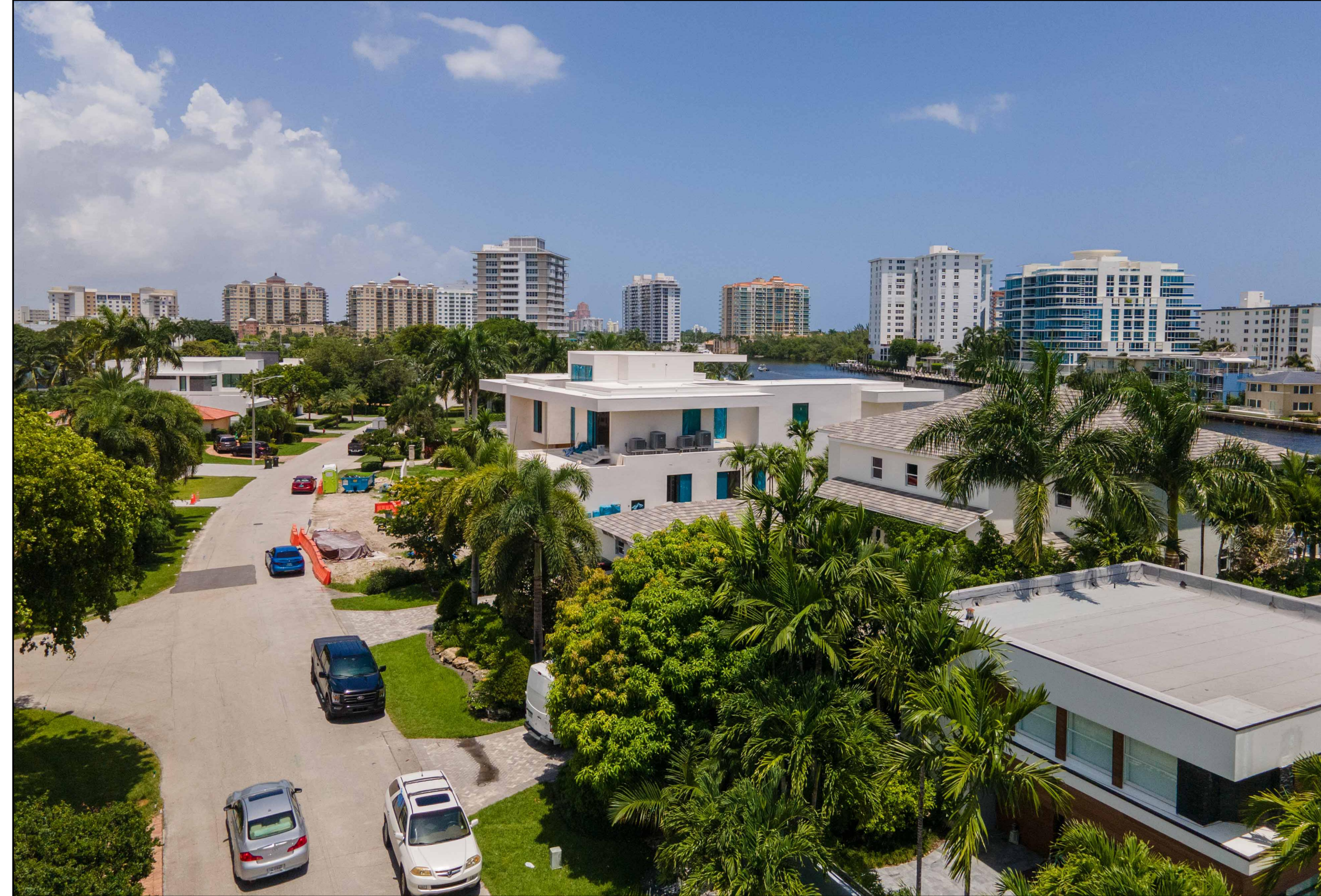
4 AERIAL VIEW #12: SOUTH-WEST SIDE, BUILDING VIEW
