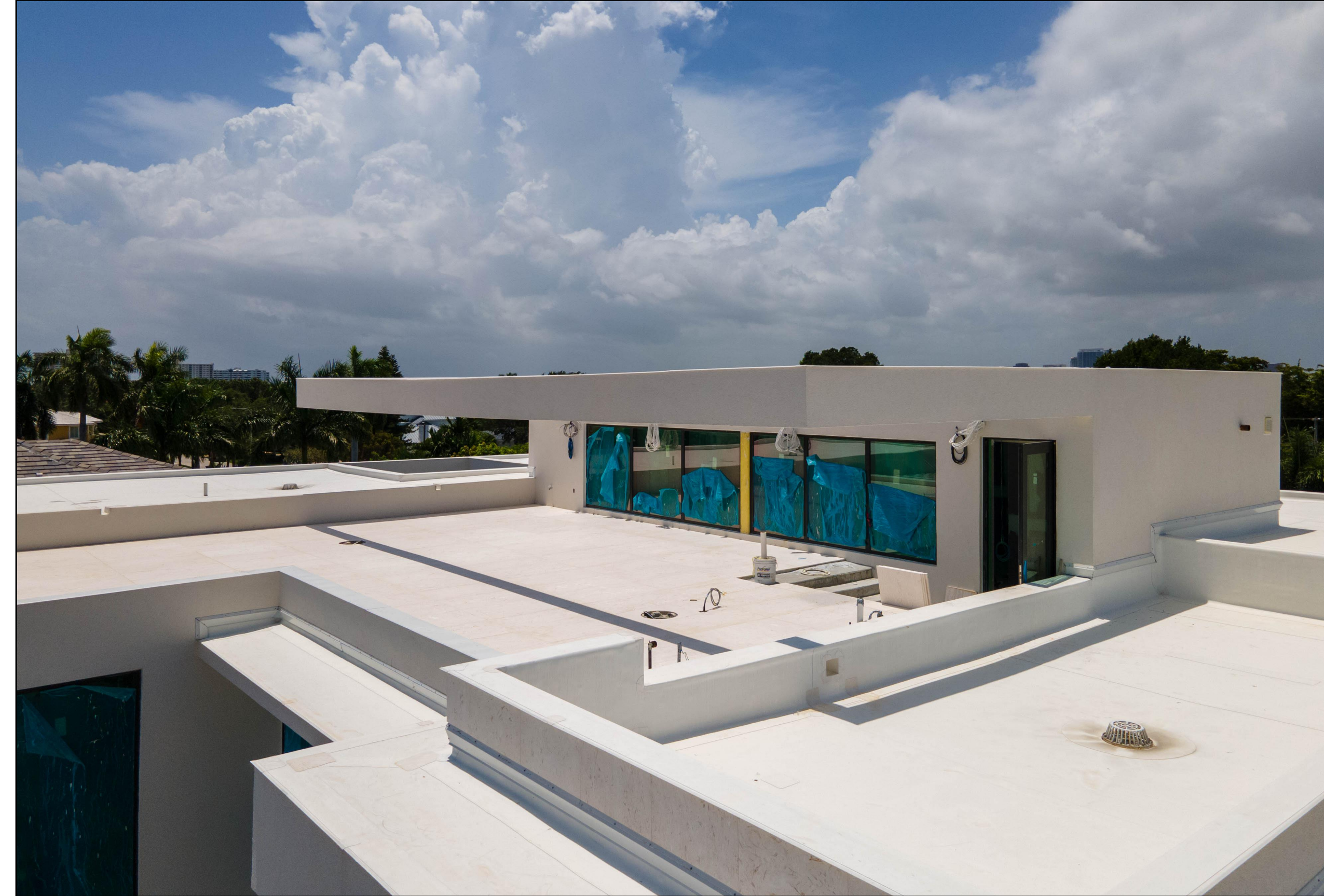
4 AERIAL VIEW #8: NORTH-EAST SIDE, ROOFTOP VIEW
