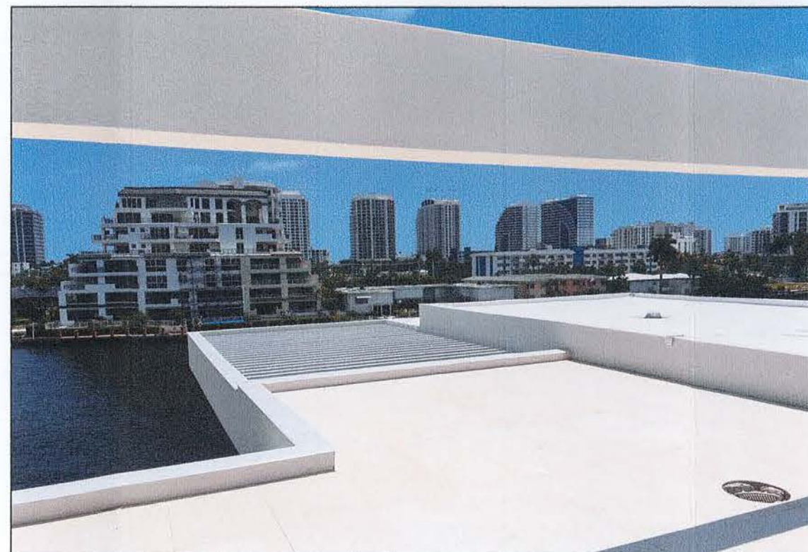
4 FIELD PHOTOS #4: ROOFTOP BEAMS FACING EAST
