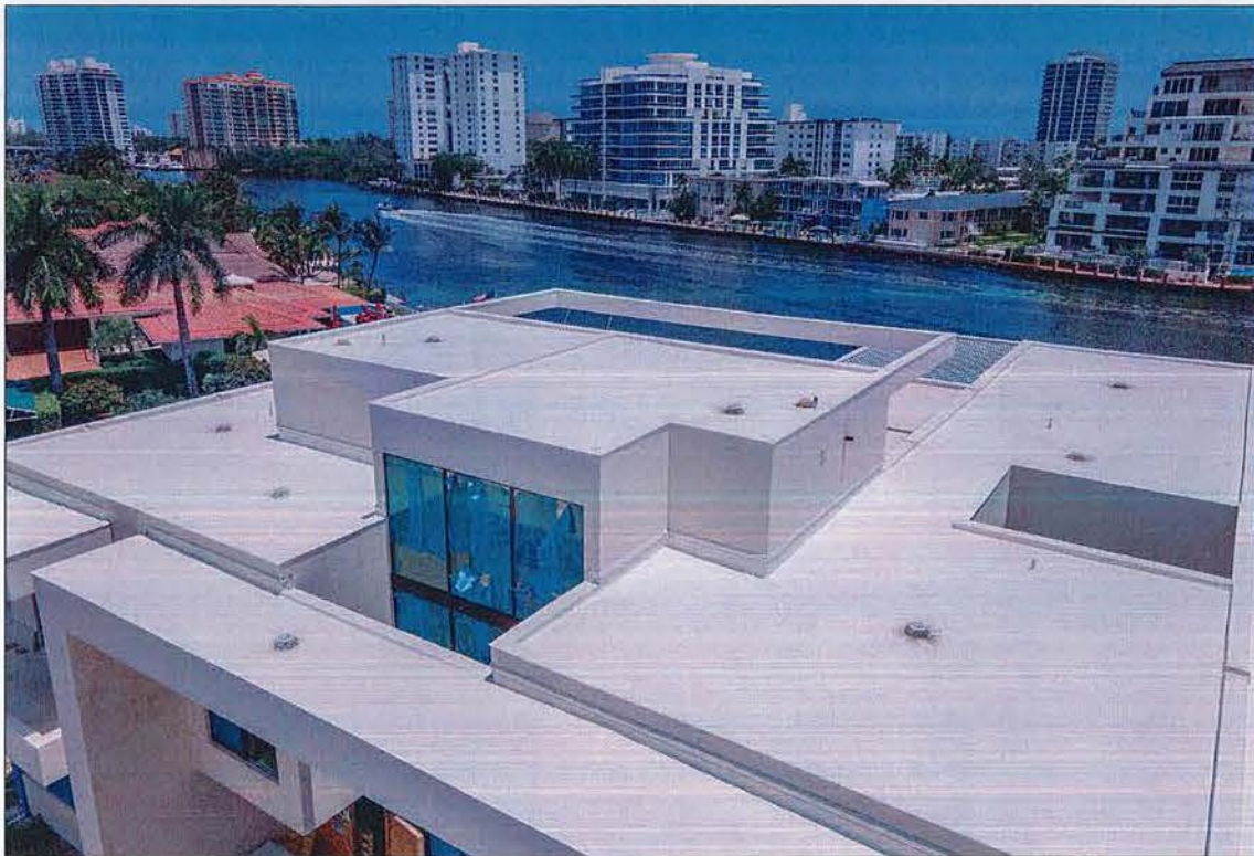
3 AERIAL VIEW #11: SOUTH-WEST SIDE, ROOFTOP VIEW Scale: N/A
