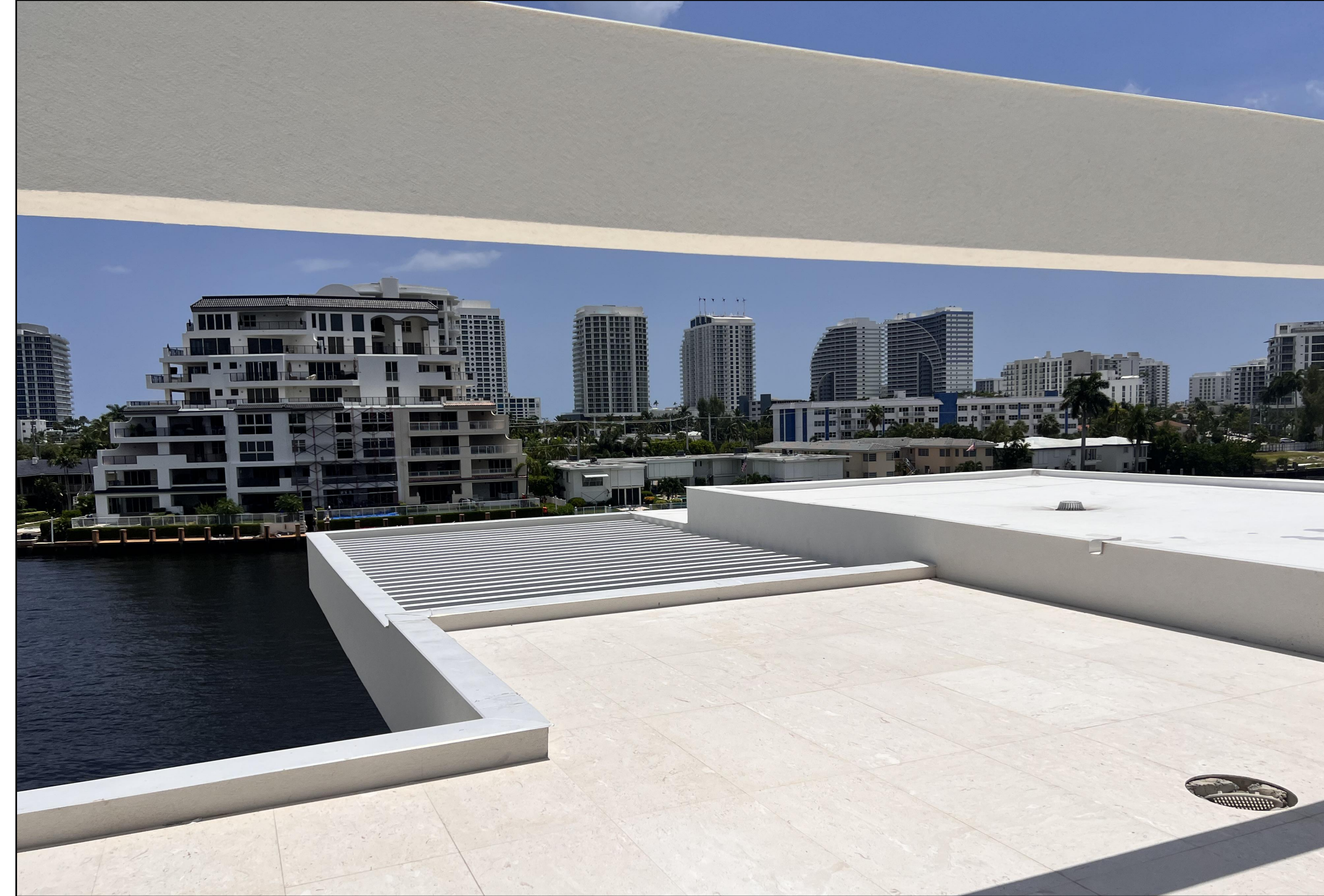
4 FIELD PHOTOS #4: ROOFTOP BEAMS FACING EAST
