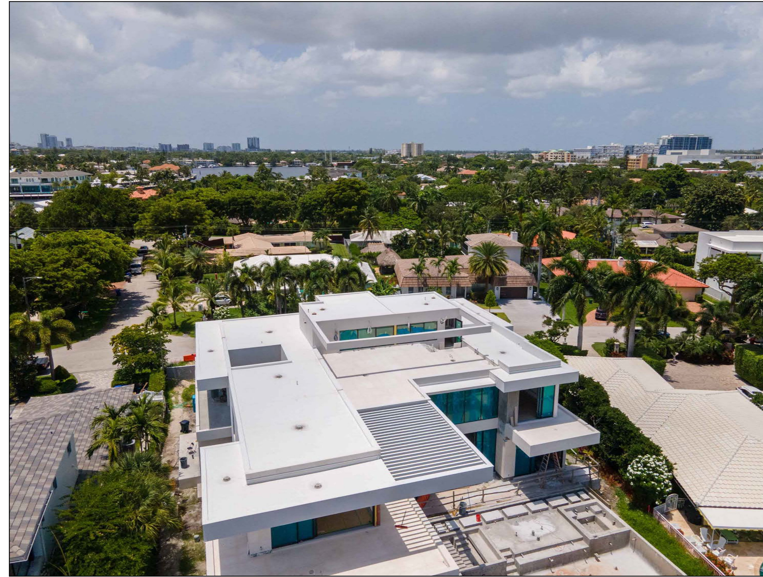
2 AERIAL VIEW #6: SOUTH-EAST SIDE, ROOFTOP VIEW
