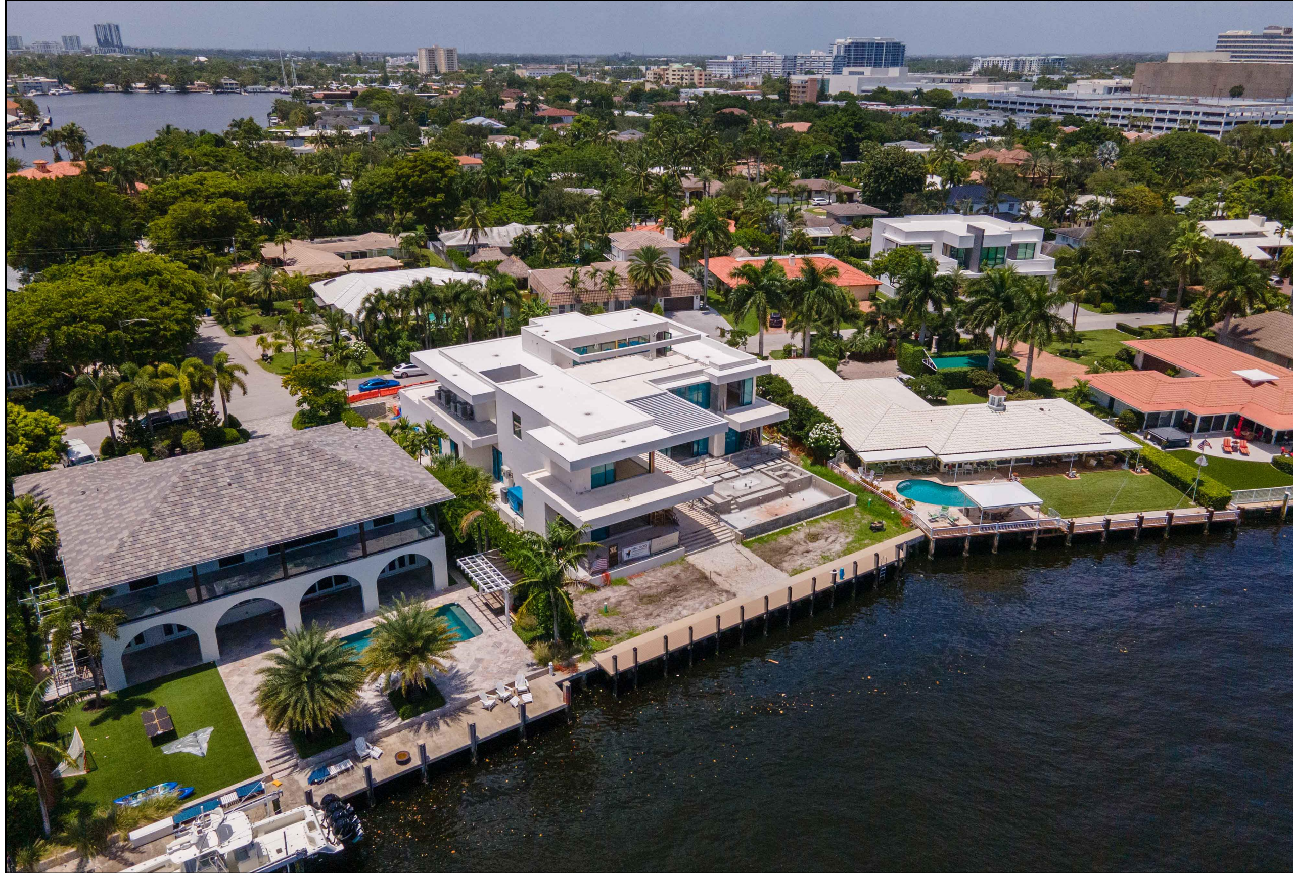
AERIAL VIEW #3: SOUTH-EAST SIDE, REAR ELEVATION
