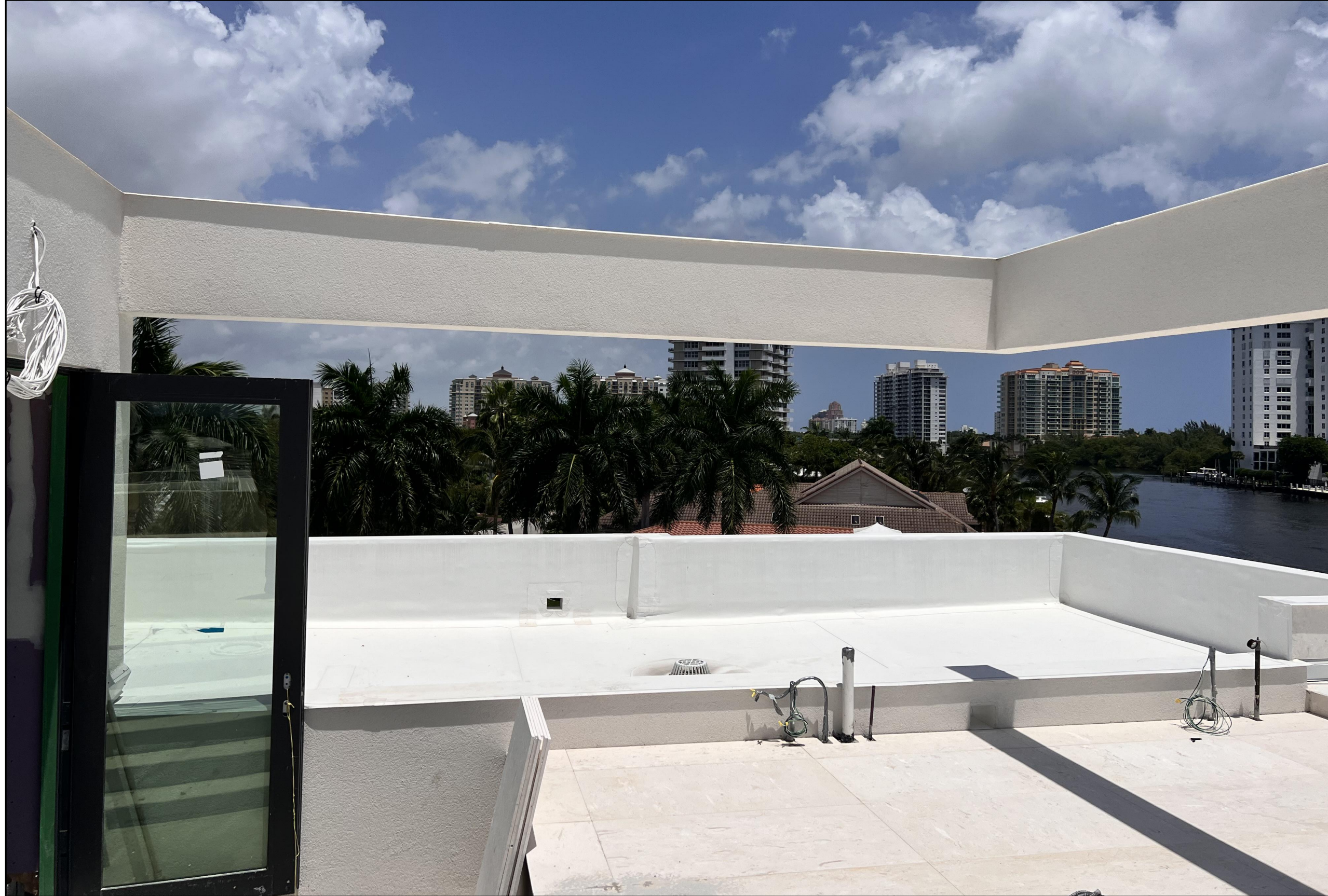
FIELD PHOTOS #3: ROOFTOP BEAMS FACING EAST
