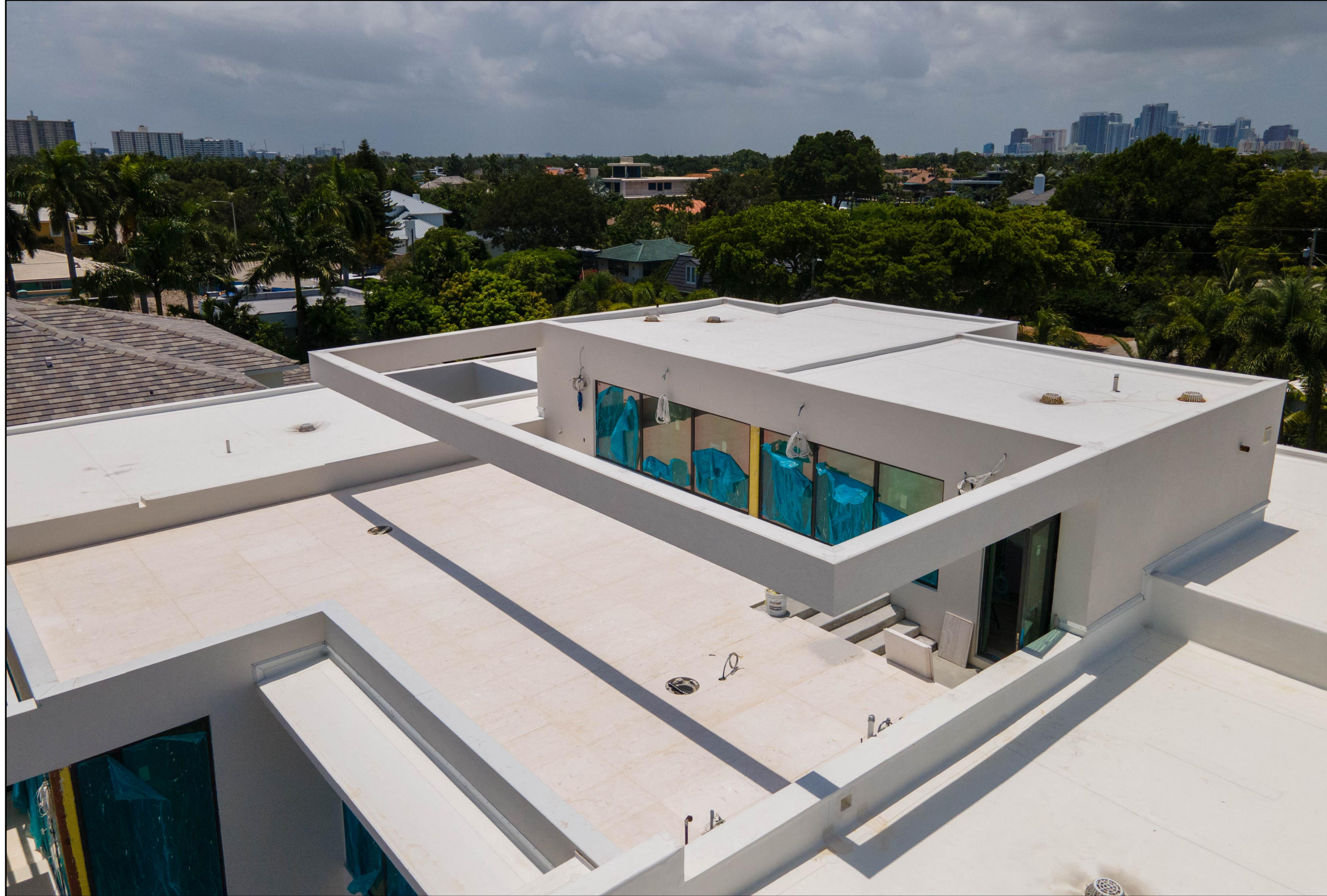
AERIAL VIEW #7: NORTH-EAST SIDE, ROOFTOP VIEW
