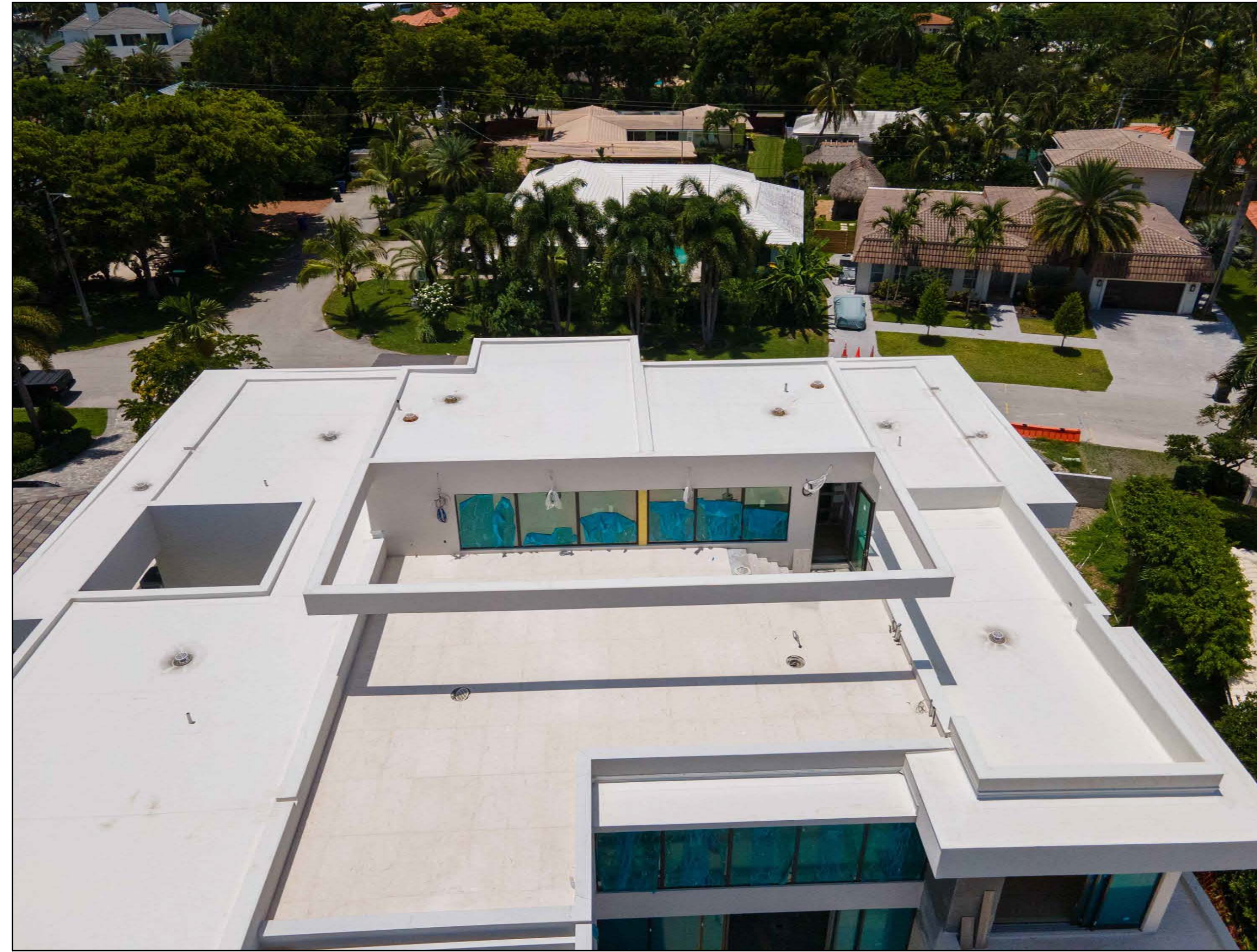
2 AERIAL VIEW #10: EAST SIDE, ROOFTOP REAR VIEW
