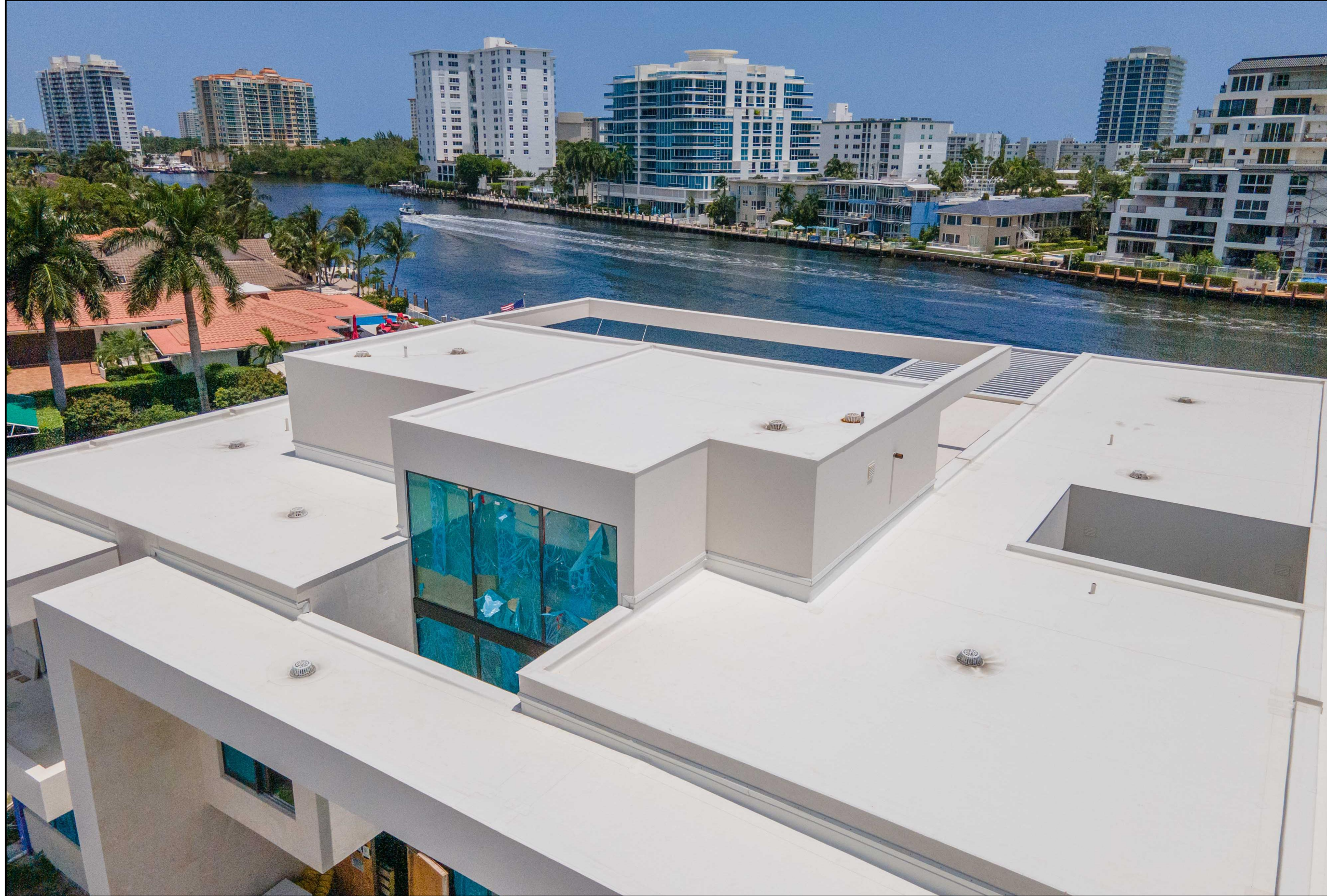
AERIAL VIEW #11: SOUTH-WEST SIDE, ROOFTOP VIEW
