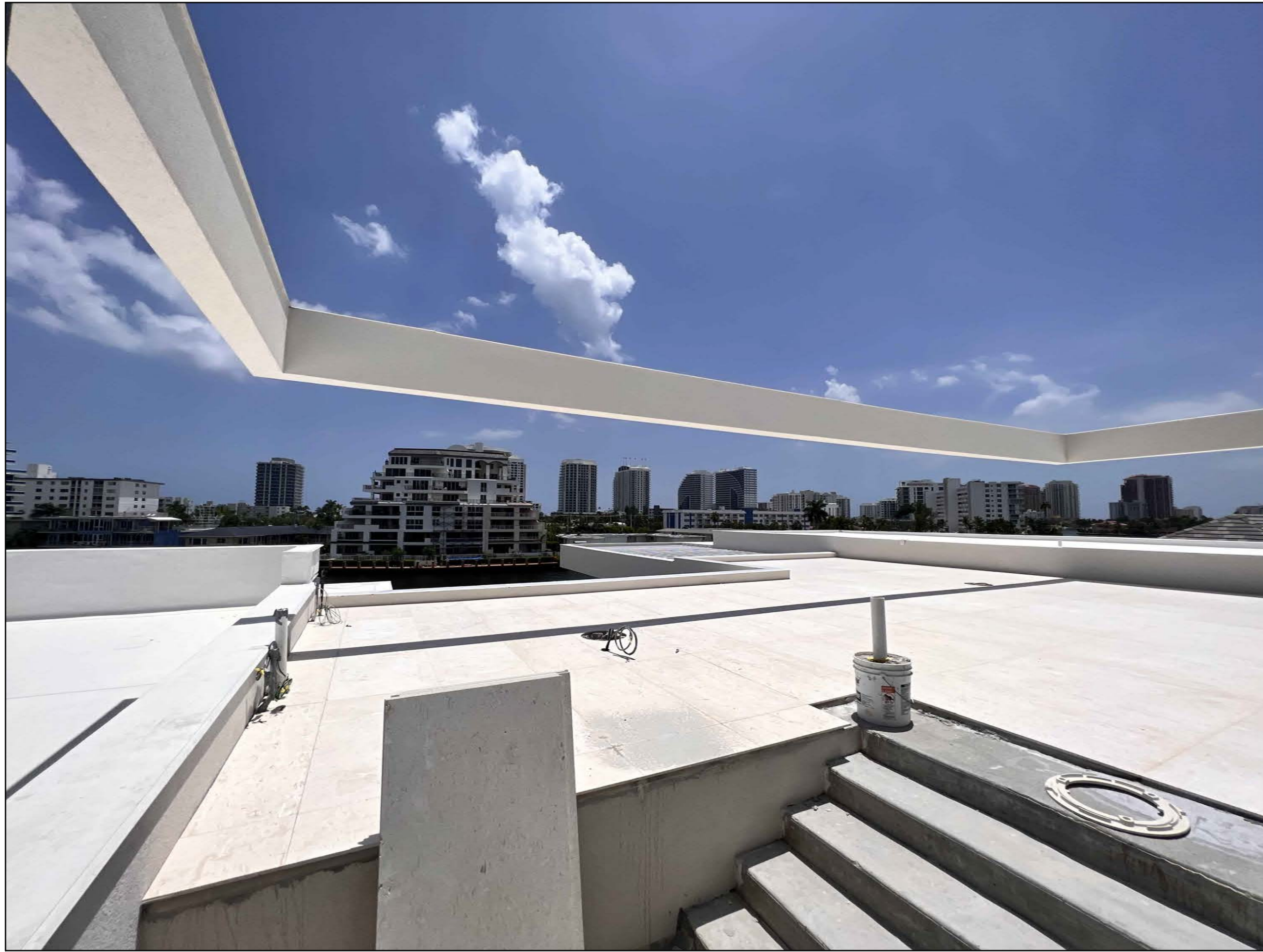
FIELD PHOTOS #1: ROOFTOP BEAMS FACING EAST
