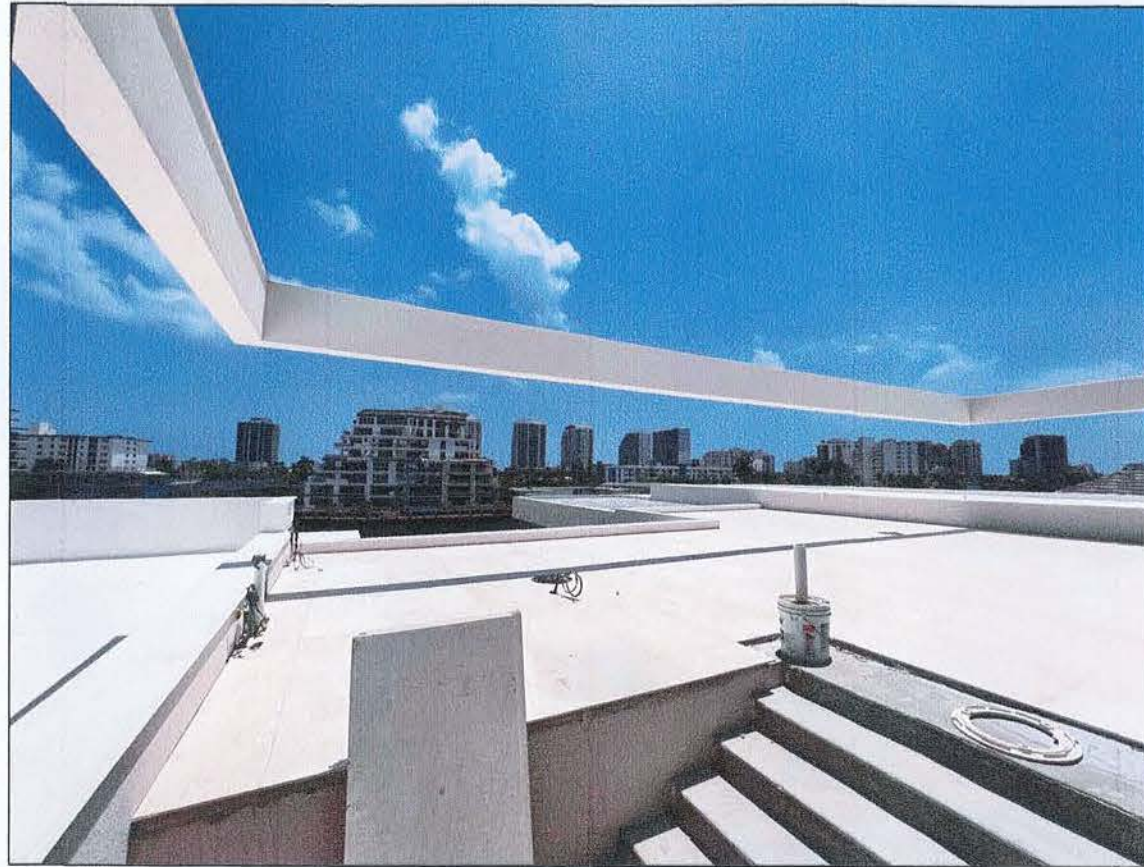
1 FIELD PHOTOS #1: ROOFTOP BEAMS FACING EAST
