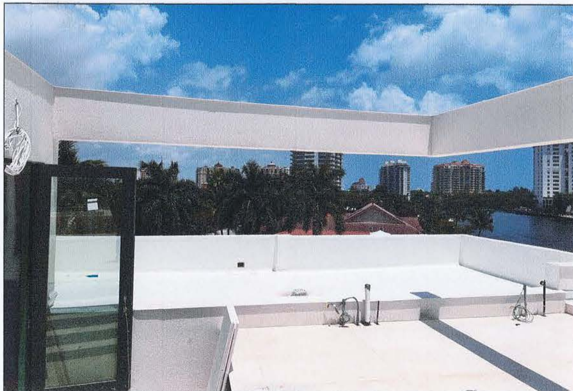
3 FIELD PHOTOS #3: ROOFTOP BEAMS FACING EAST
