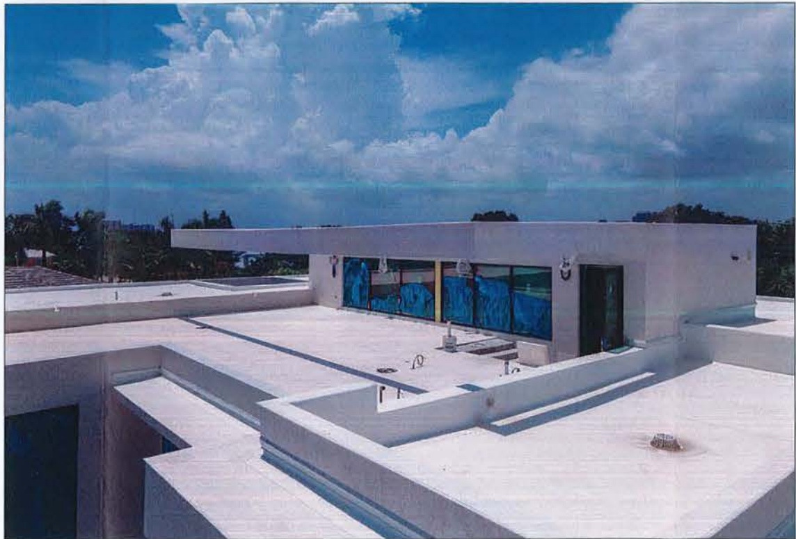
4 AERIAL VIEW #8: NORTH-EAST SIDE, ROOFTOP VIEW
