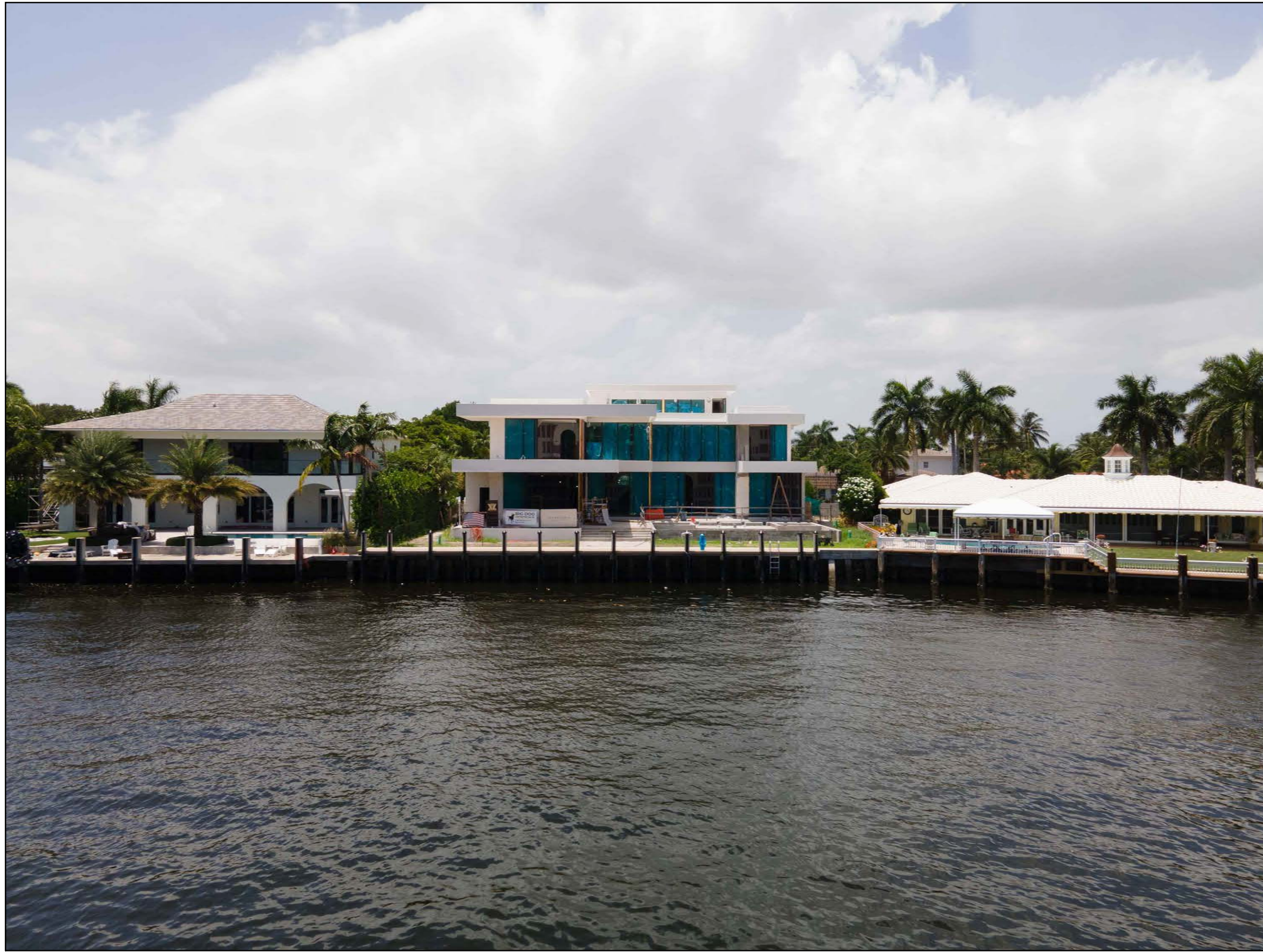
AERIAL VIEW #5: EAST SIDE, REAR ELEVATION
