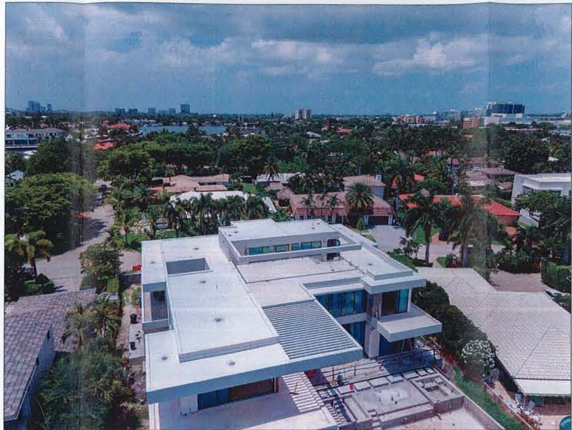
2 AERIAL VIEW #6: SOUTH-EAST SIDE, ROOFTOP VIEW
