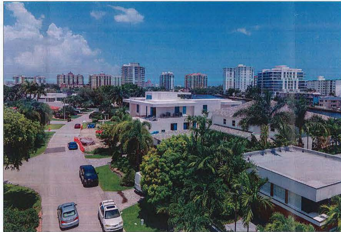
4 AERIAL VIEW #12: SOUTH-WEST SIDE, BUILDING VIEW Scale: N/A
