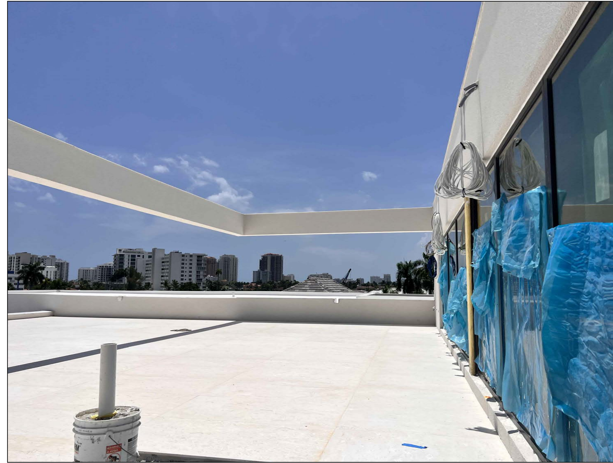
2 FIELD PHOTOS #2: ROOFTOP BEAMS FACING EAST
