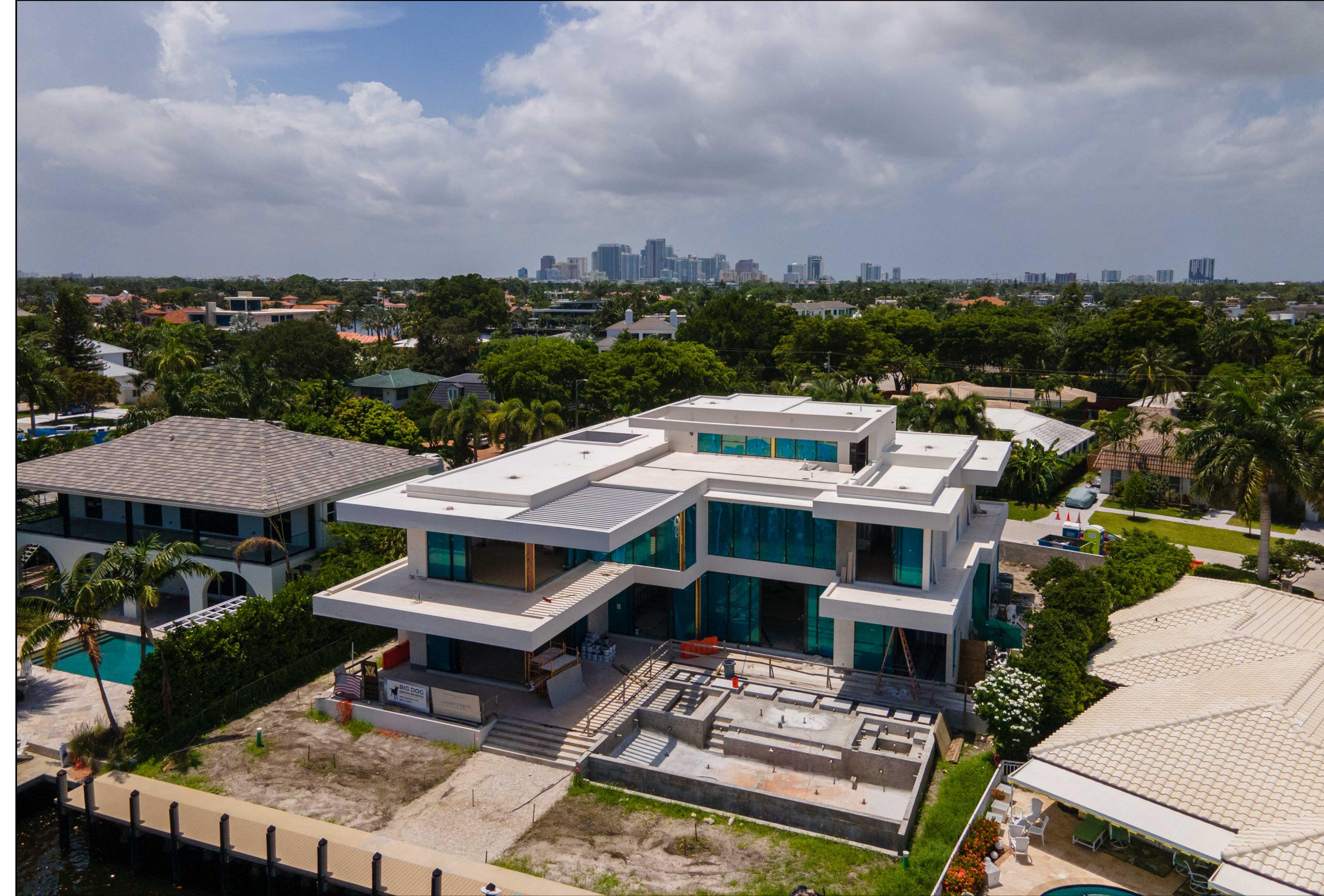
4 AERIAL VIEW #4: NORTH-EAST SIDE, REAR ELEVATION
