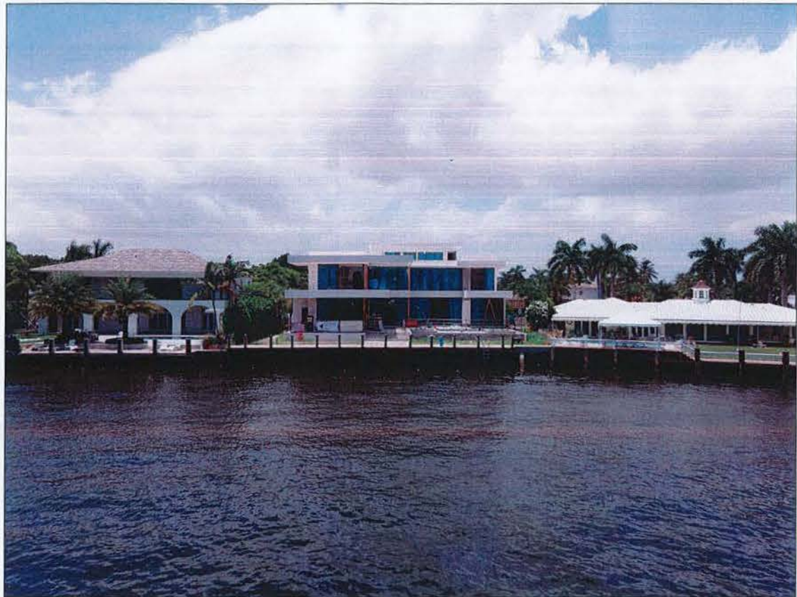
1 AERIAL VIEW #5: EAST SIDE, REAR ELEVATION
