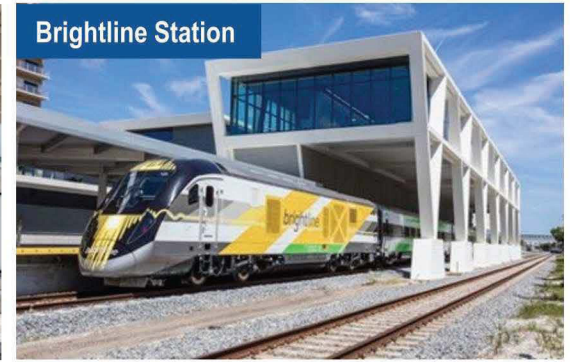
Existing Intercity Passenger Rail Station
