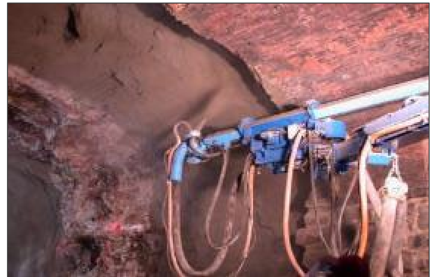
Figure 30: Construction During SEM Example 2
