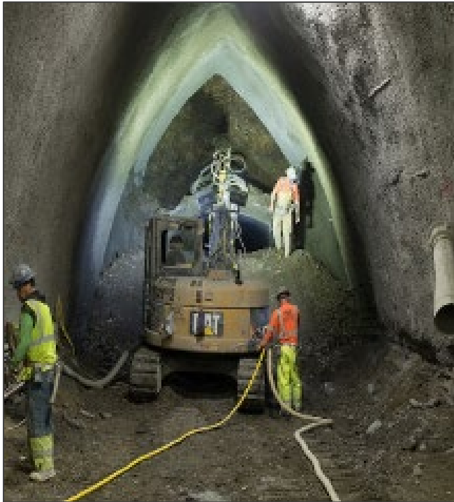
Figure 33: Construction During SEM Example 3
