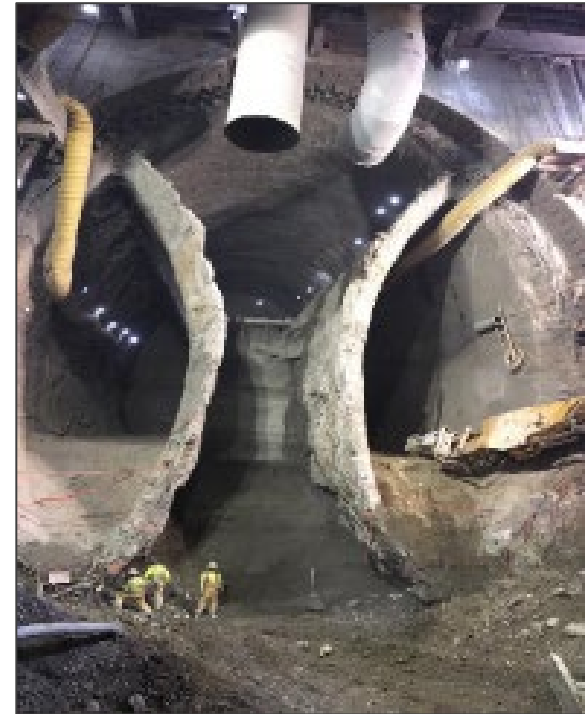
Figure 32: Construction During SEM Example 4
