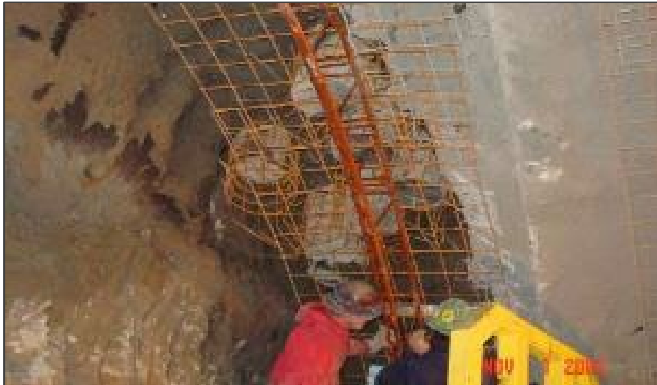
Figure 31: Construction During SEM Example 1
