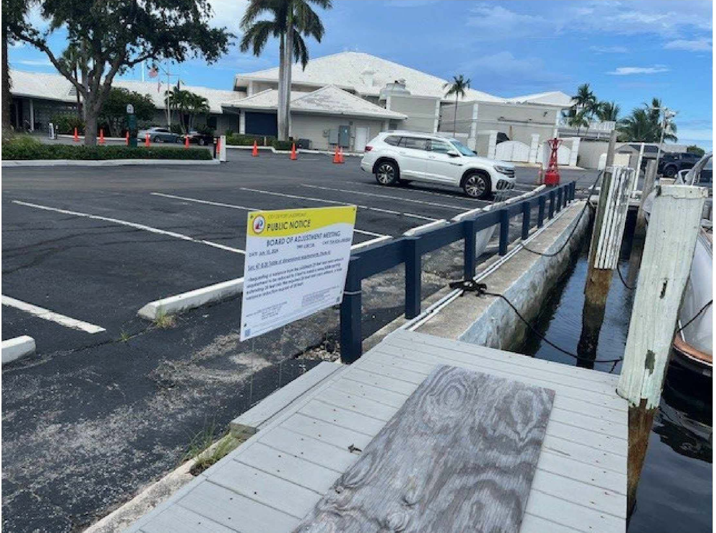
1. South view of site from waterway.
