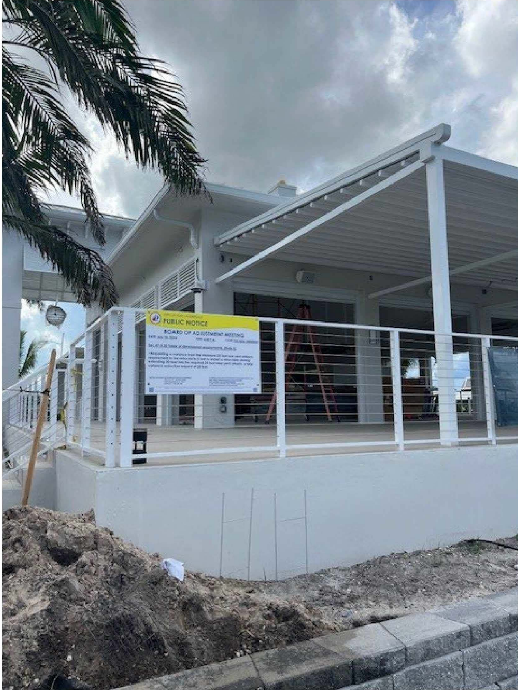
4. East view of site from waterway.
