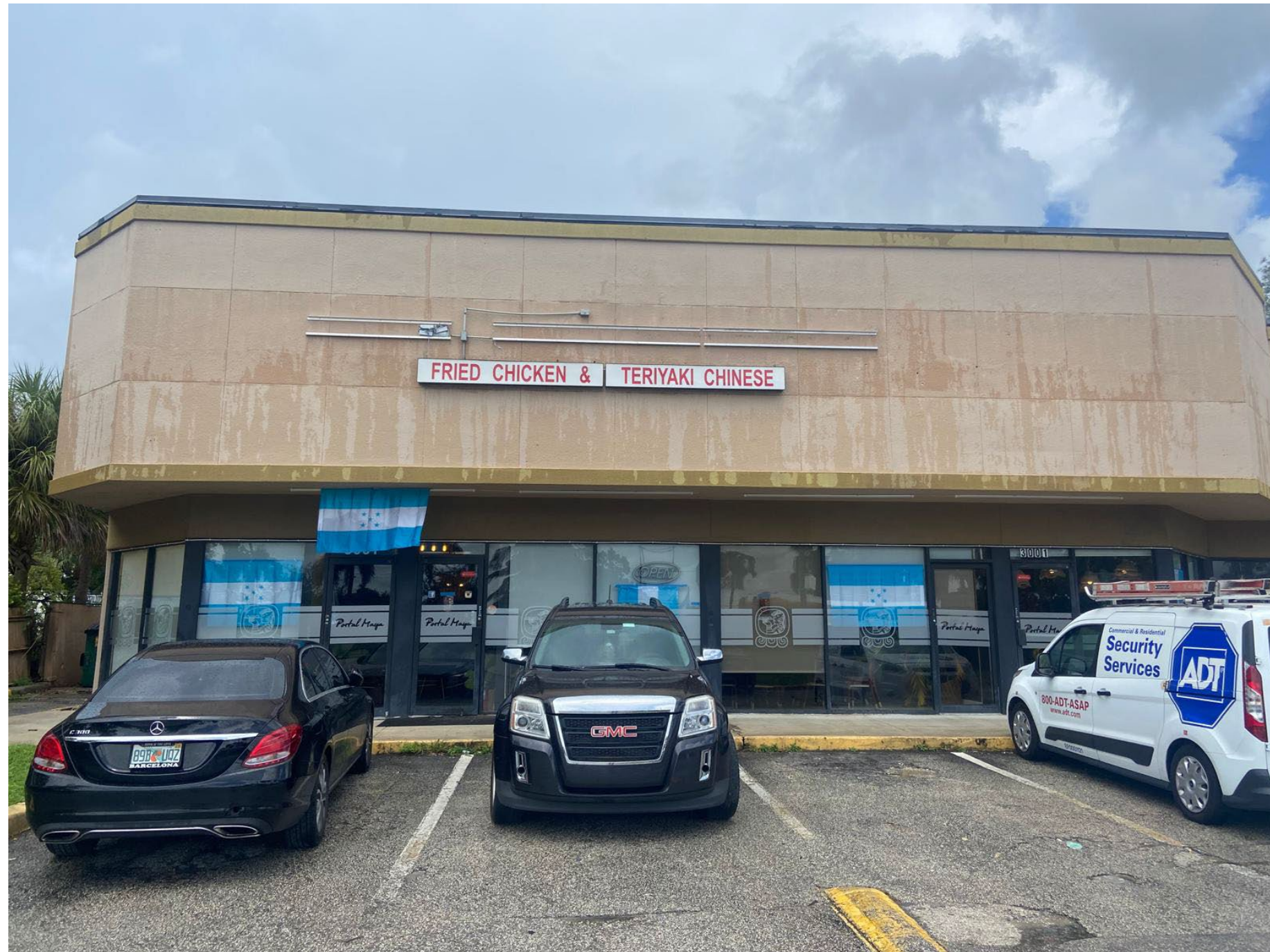
Exterior Under Renovation
